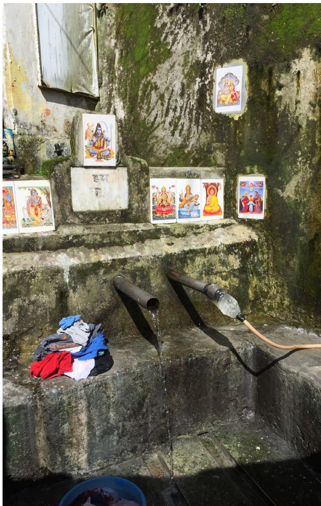
Public water pipes in Gangtok, India. Credit: David Dodman
